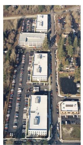
The Tigard Corporate Center consists of three two-story architecturally designed concrete tilt buildings, each with a steel structural system and Class A core and office interiors. In addition, a 362-stall, 5-story parking garage was built for Household International, who leased the entire complex during the construction phase of the project.
